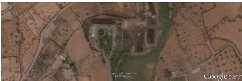
Figura 2: PTAR de Ouardanine (Google Earth, 2015)
