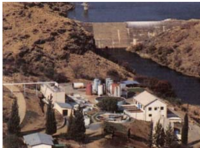
The Goreangab Dam, adjacent to the Windhoek reclamation plant in Windhoek, Namibia. Photo courtesy of Valentina Lazarova
