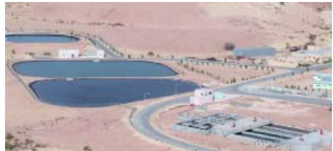
Wadi Musa secondary treatment plant and storage ponds serving communities in the vicinity of Petra, Jordan. Photo courtesy of Bahman Sheikh
